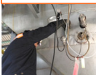
Flue Gas Temperature and Compositions Measurement
